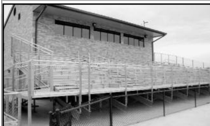
Track & Field Complex
